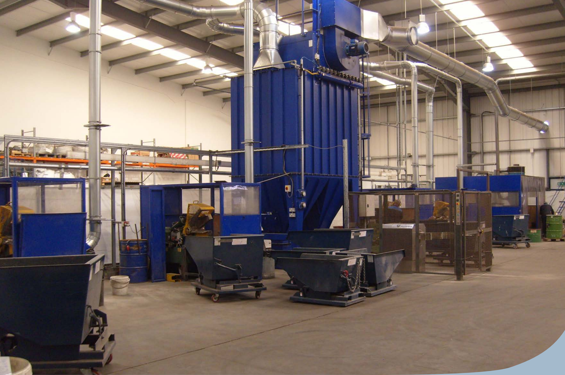
PRL's modern facilities dedicated to the recycling of auto-cats
